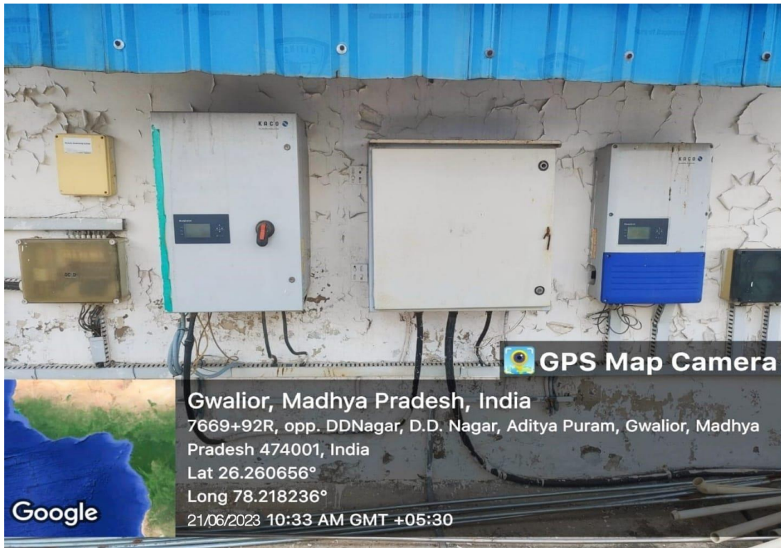
Rooftop solar panel system in Block A
