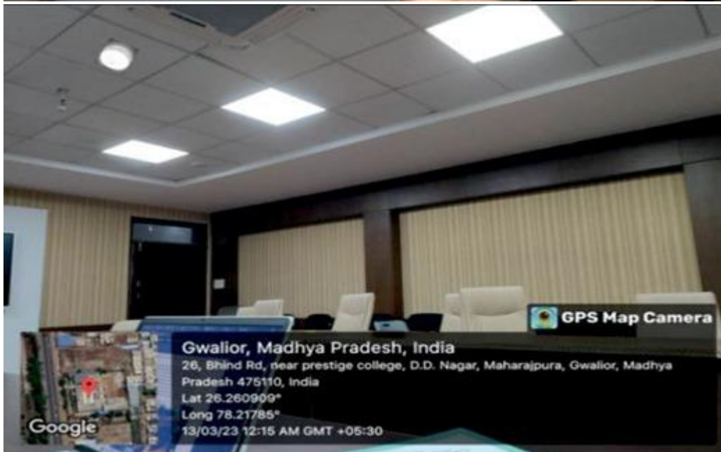
Solar sensor system in Board Room
